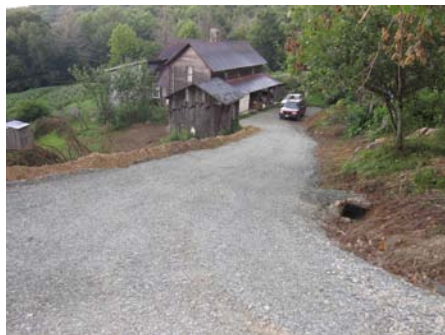
Hicks Driveway - Completed
