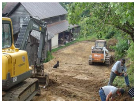
Hicks Driveway - Work in Progress
